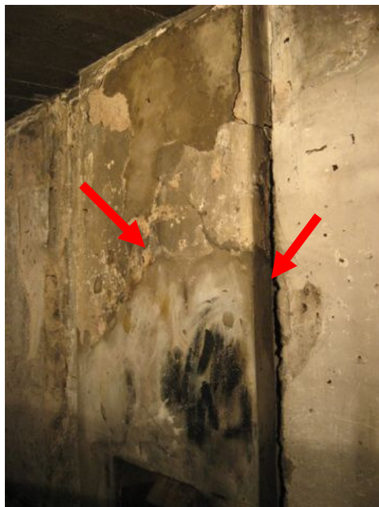
Photo 11 – Chimney breast moving away from party wall
