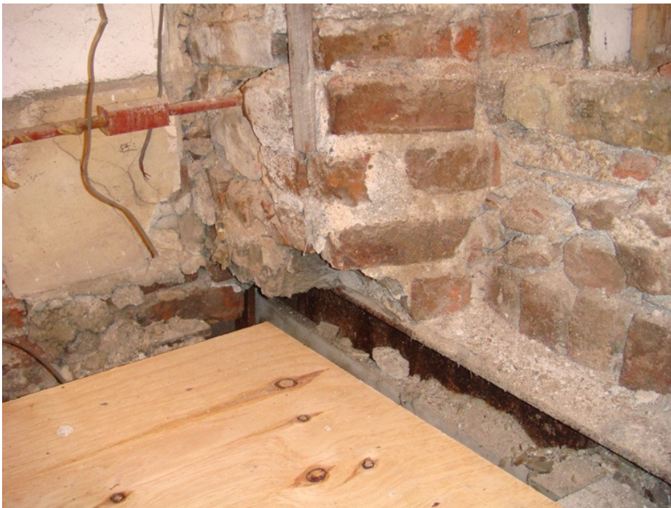
Photo 26B – Erosion of support to masonry at window reveal
