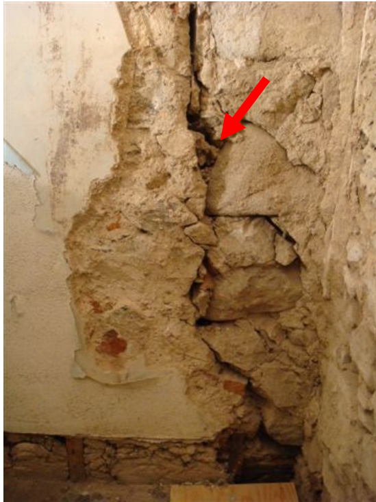
Photo 23 – Vertical crack in the original rear wall
