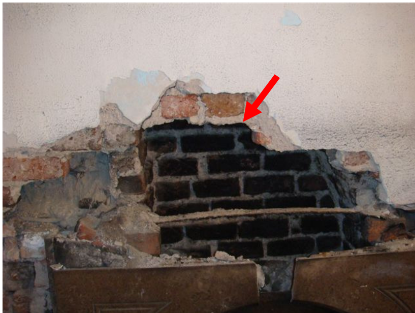
Photo 22 – Disruption in masonry over chimney breast
