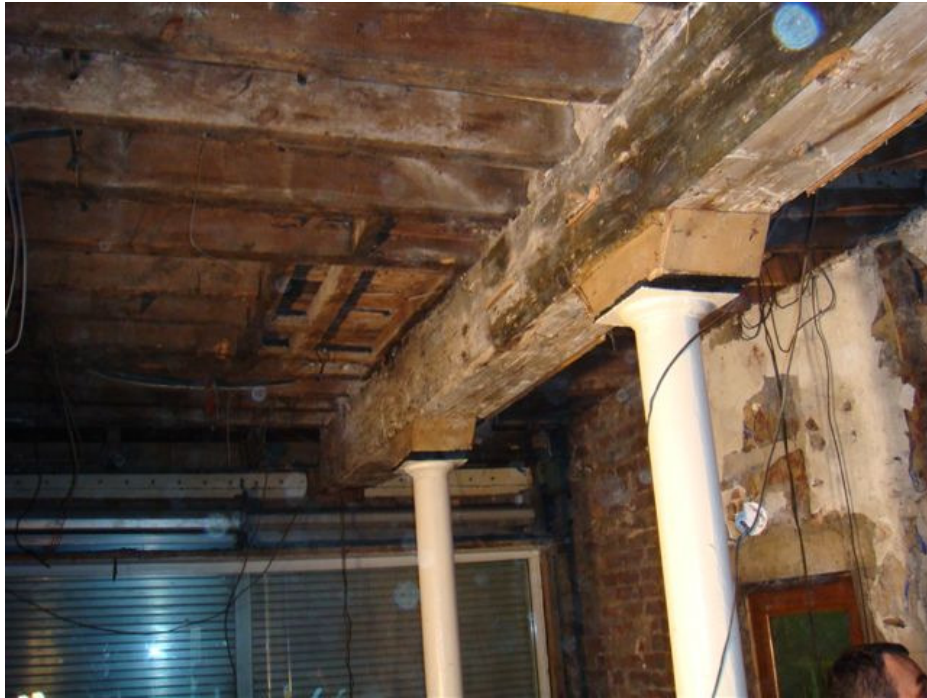
Photo 35A – Timber beam support for the intermediate wall
