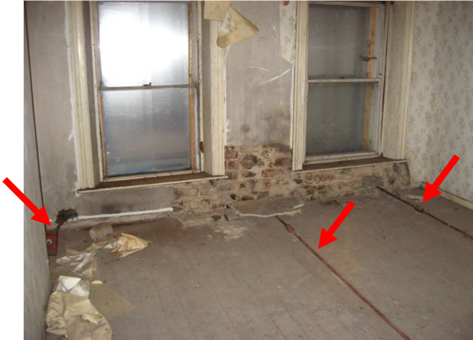
Photo 12 – 2 nd Floor bedroom 1 tie rods
