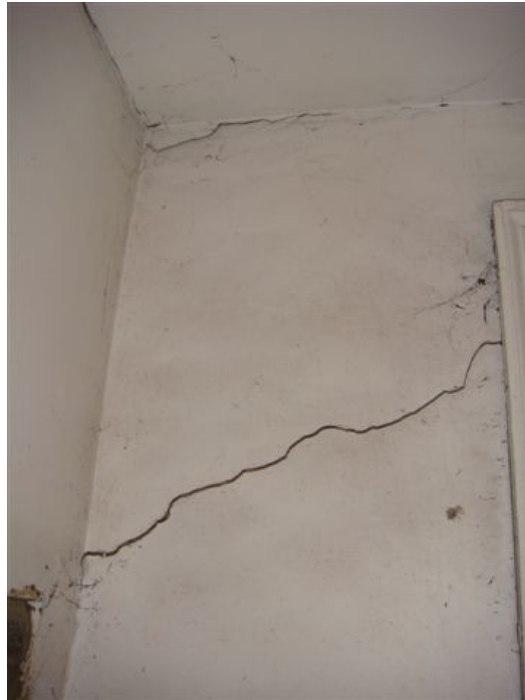
Photo 16 – Diagonal crack approx. 3-4mm wide
