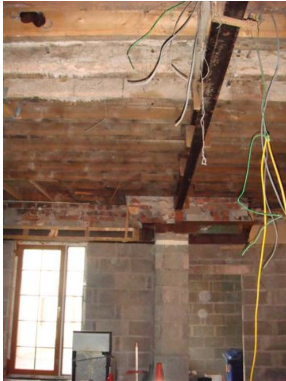
Photo 31 – 1 st floor steel beam support
