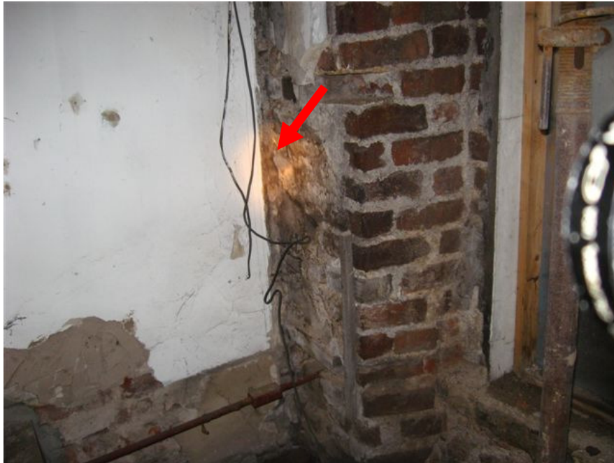
Photo 26A – Gap between intermediate wall and the front façade
