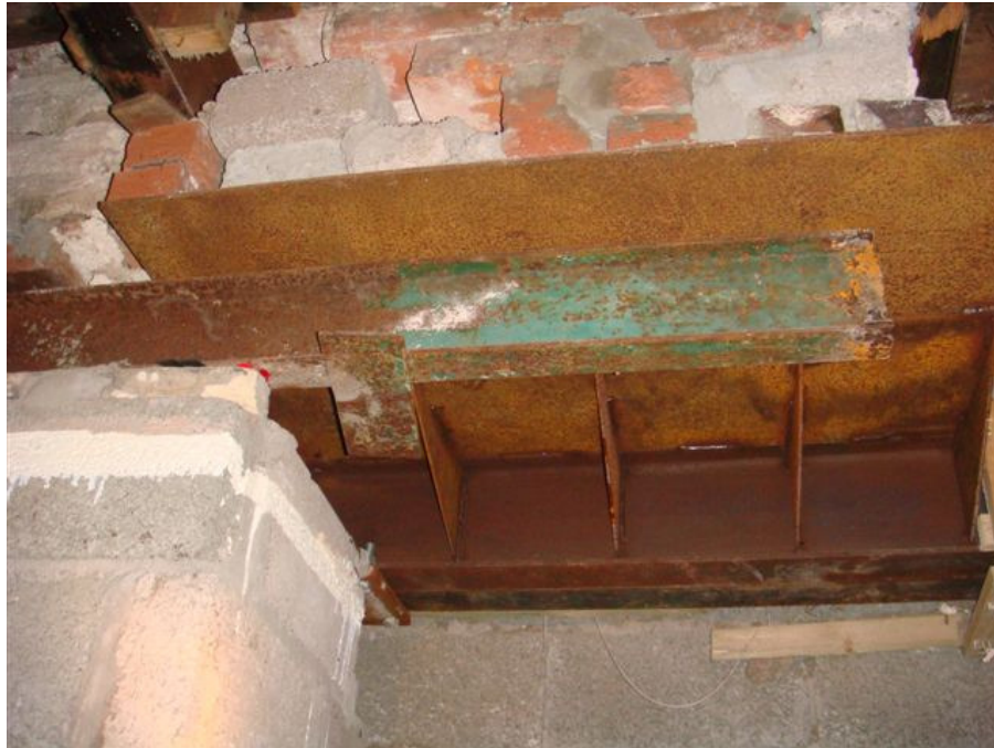
Photo 33 – Support arrangement for rear chimney
