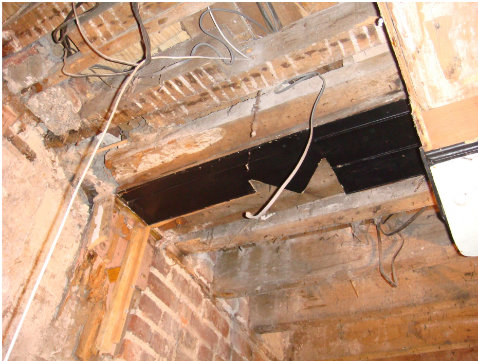
Photo 34C – Rot to end of timber beam at external wall to alley
