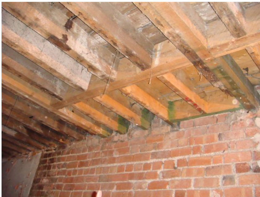
Photo 30 – 1 st Floor joists cut & spliced with binder
