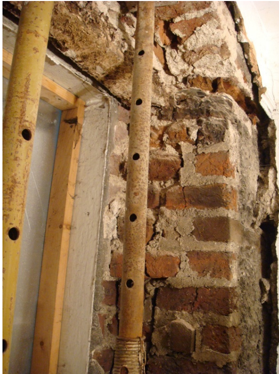
Photo 29B – Disruption to masonry at head and reveal of window
