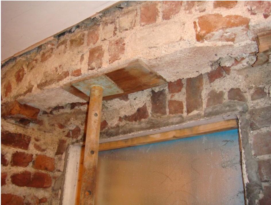
Photo 26B – Complete loss of timber head
