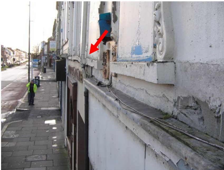
Photo 43 – Unevenness in 1 st floor sills
