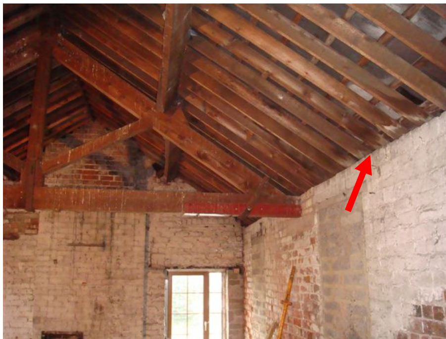
Photo 5 – Damp and rot at rafter support on party wall
