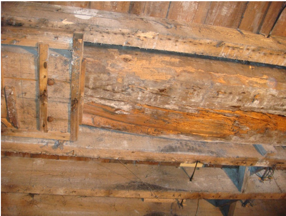
Photo 35B – Rot to underside of timber support beam
