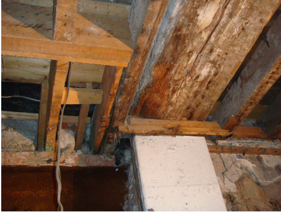
Photo 34B – Rot to end of timber beam at support
