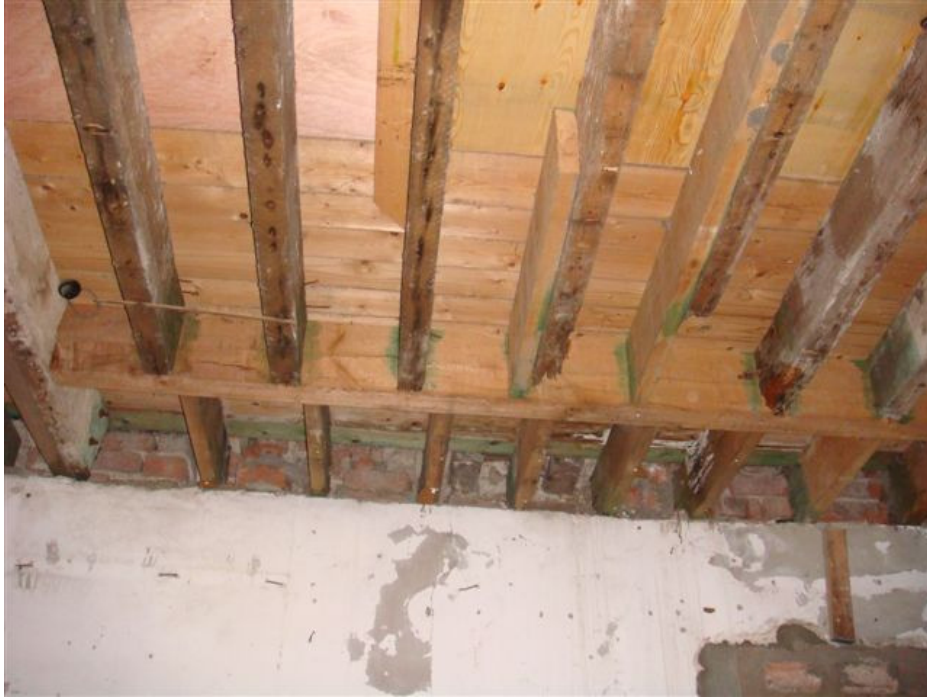
Photo 7A – 2 nd floor joists cut & spliced on binder
