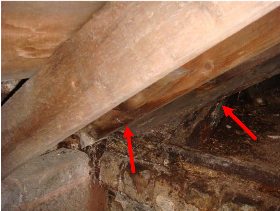
Photo 4 – Damp and rot in the existing building rafters
