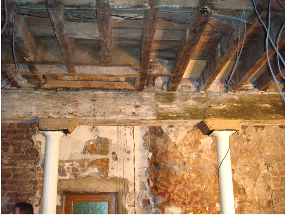
Photo 36A – Timber beam supporting the intermediate wall.
