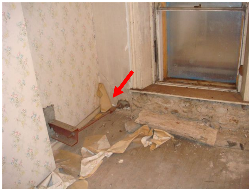
Photo 15 – Diagonal crack above the tie rod
