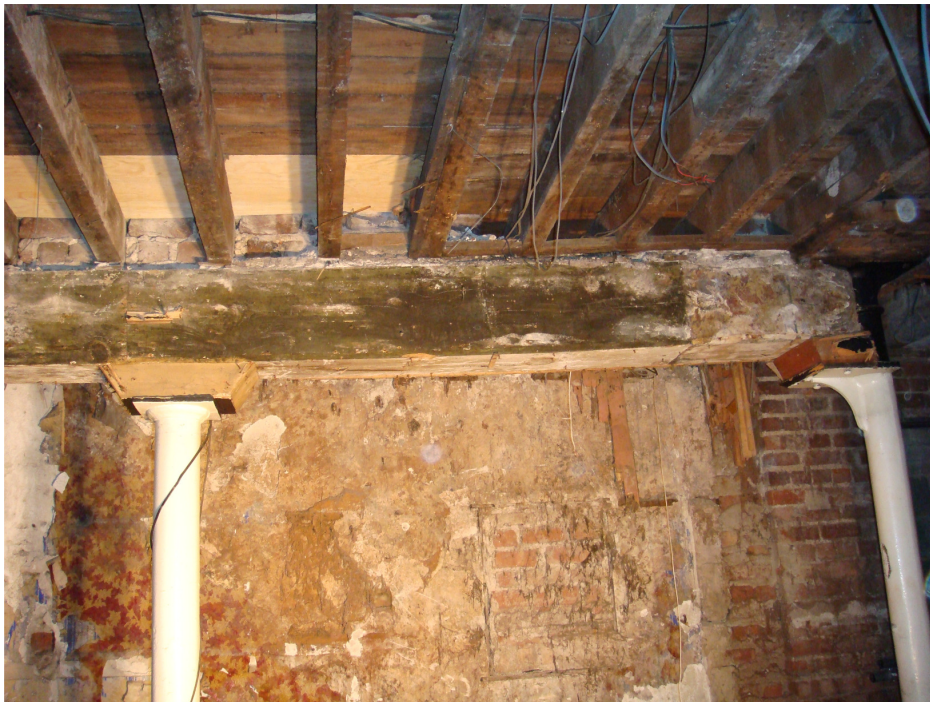
Photo 36B – Deflection in timber beam and rotation of support
