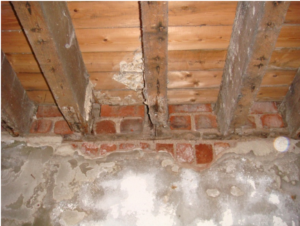
Photo 7B – Damp & rot in 2 nd floor joists along the party wall
