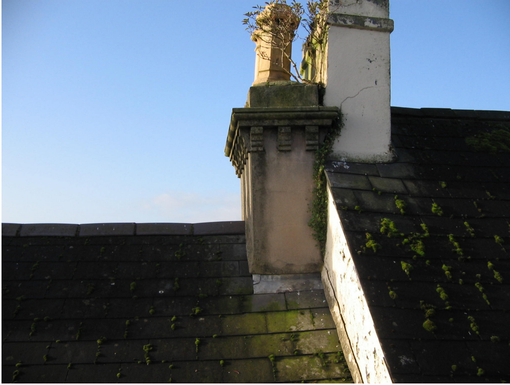
Photo 44 – Disruption to chimney and party wall at roof juncture.
