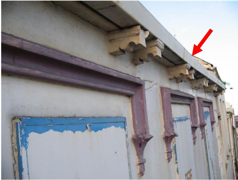
Photo 40 – Unevenness in gutter line
