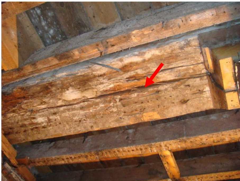
Photo 34A – Split in timber beam supporting original rear wall.
