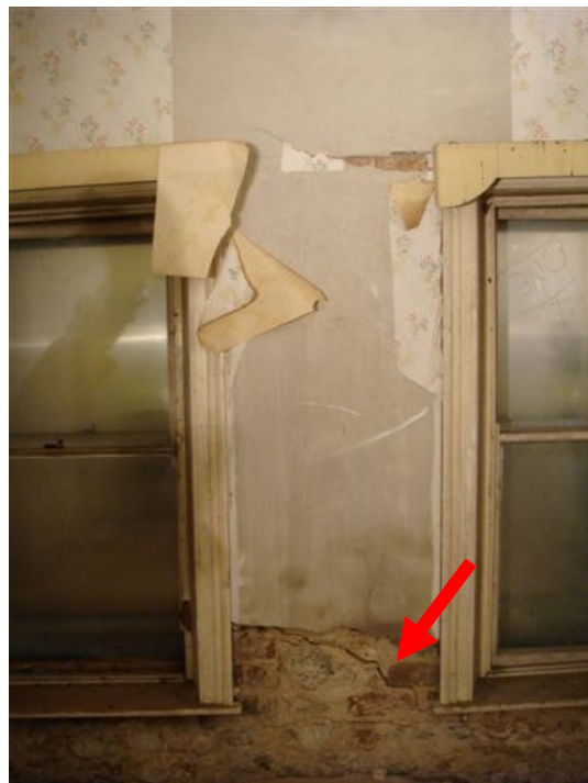
Photo 13 – Diagonal crack approx. 3-4mm wide between windows
