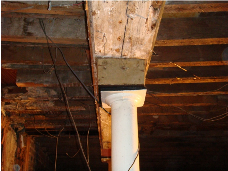
Photo 36C – Decay in adjacent joists and poor support alignment
