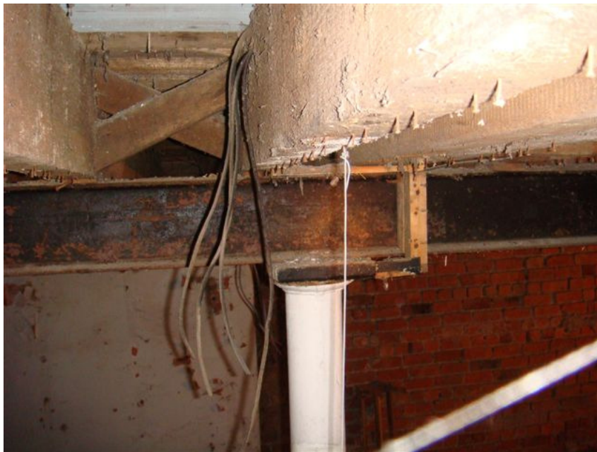
Photo 32 – Post support of the 1 st floor steel beam
