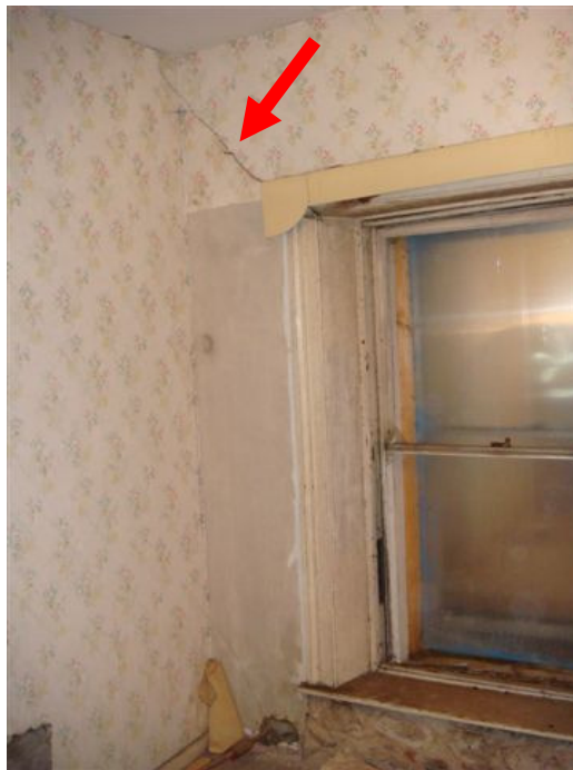
Photo 14 – Diagonal crack above window
