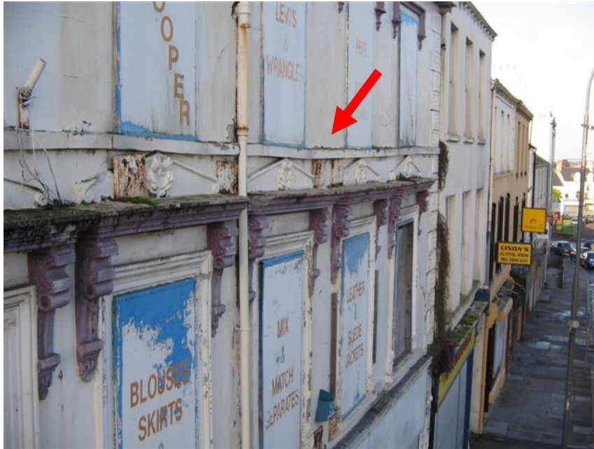
Photo 42 – Unevenness in 2 nd floor sills
