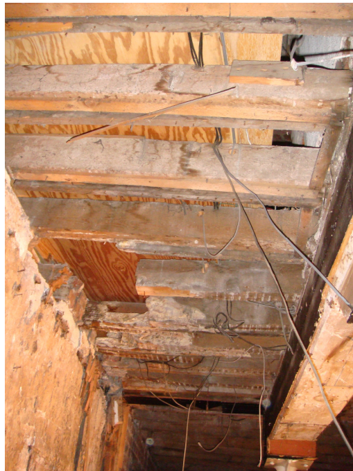
Photo 36D – Close up of decay and disruption to joists
